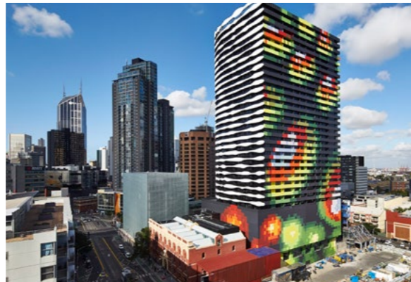
CUB building with the apartment (Image Ref. 8)
